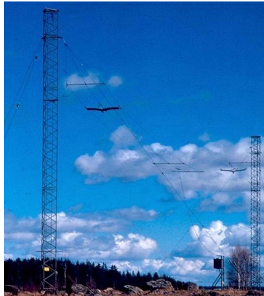
Bredbandsdipol 2 – 9 MHz 10 kW
